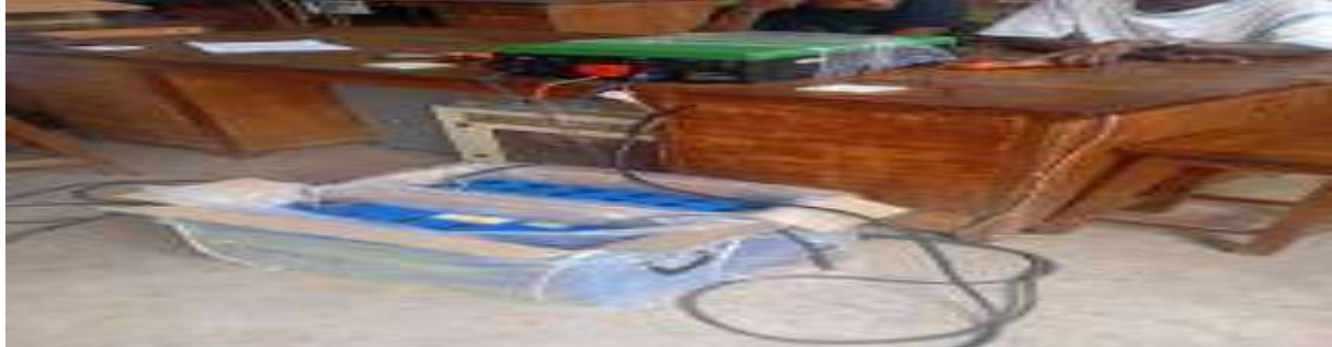
Fig. 1: Experimental set up of 5.2 kVA, 24V hybrid inverter
